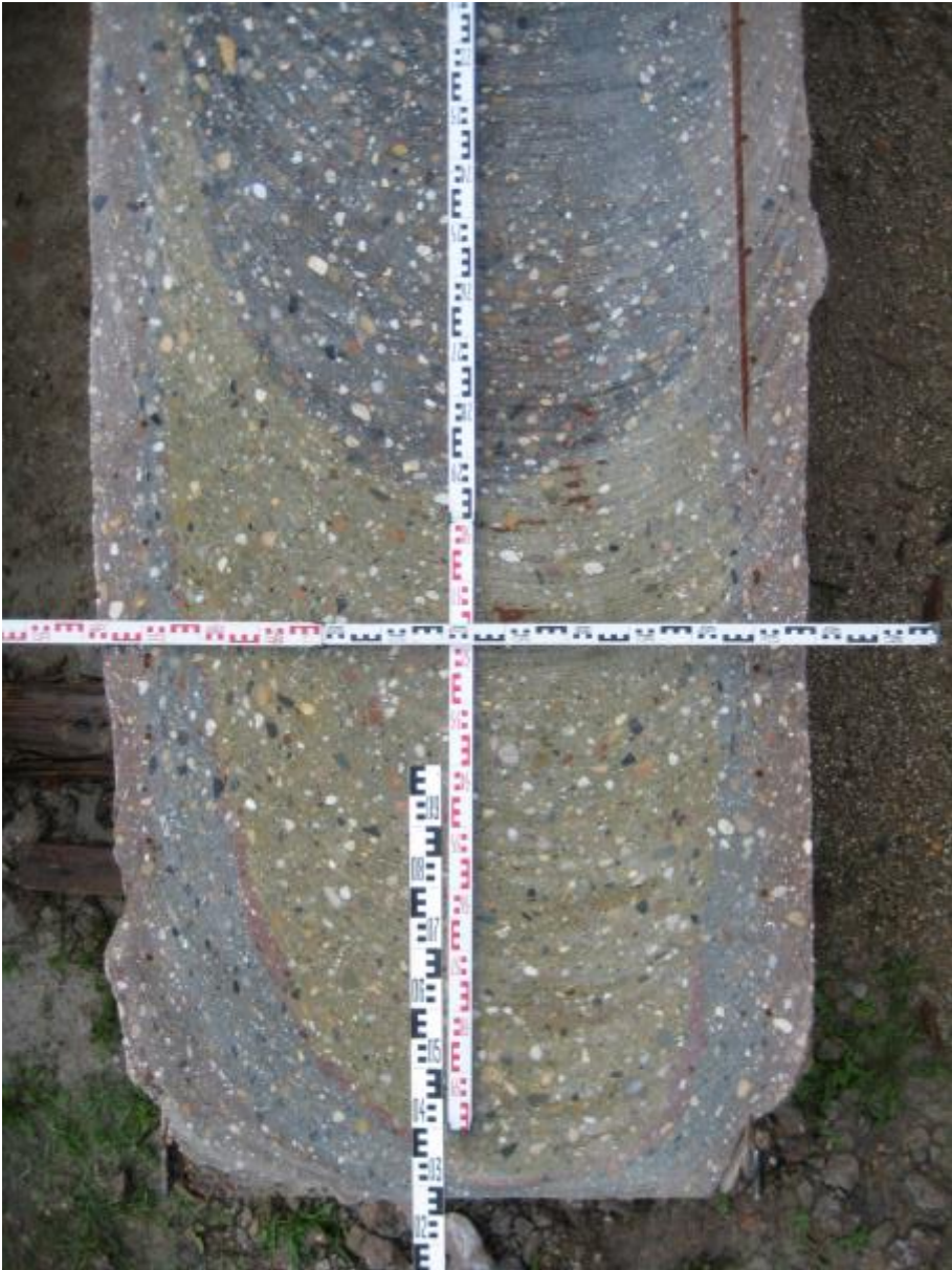
FIGURE 6.3 – Cross section of a bored pile cast with differently dyed loads of tremie concrete
