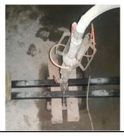
Action Taken, Lessons Learnt: An analysis was carried out and found: It is recommended to secure the nozzle with additional safety devices after anchoring. Additional anchorages of the nozzle. Chain to secure the hose. All work near the pressing nozzle only after the pressing process has been completed.
