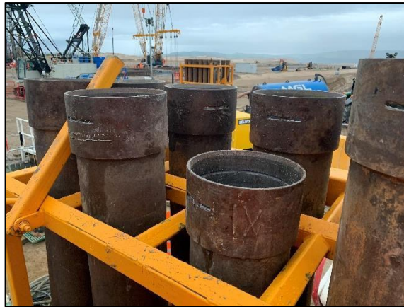
Lead tremie placed in tremie rack after the incident. The collar had been 100mm lower during the incident.
