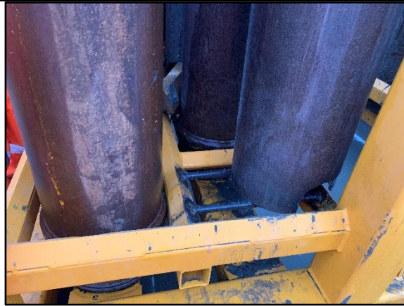
Modification made to tremie rack to accommodate the lead tremies.
