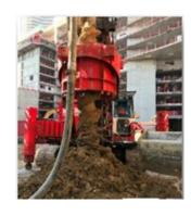
A crew was performing an operation in an area where old anchorages were located. During drilling, the auger hit an old buried anchorage (not identified on the drawings) that got twisted on the auger. Once the drilling was completed, the tool is gradually raised (concreting phase). When the foot of the auger came out, the tensioned anchorage is abruptly unrolled, sweeping a 4m radius around the auger, almost hitting personnel, who were however standing outside the machine's restricted zone
