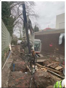
Action Taken, Lessons Learnt: Setting the work. Creation of a load-bearing working level or cover. Adjustment of planning / relocation of pile installation points, if necessary. Carrying out safety briefings before starting work.
