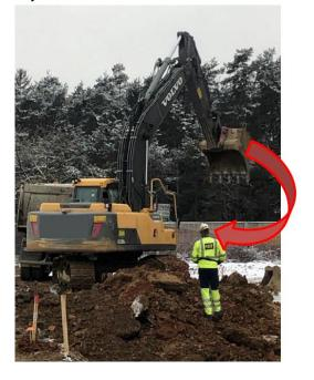
Action Taken, Lessons Learnt: Do not stay in the danger zone during dredging. Access to the danger zone only after clear contact with the machine operator and setting of the excavator. Determination of measures based on the findings of the evaluation Field of vision with restricted field of vision. Instruct the employees. Close off the danger zone. Retrofitting of camera systems. If necessary, call in a banksman.
