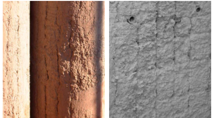
FIGURE D.5 SHADOWING IN A PILE (LEFT); MATTRESSING IN A PANEL (RIGHT)
