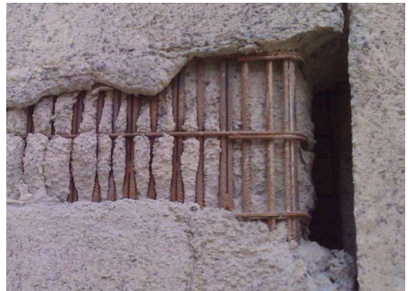
FIGURE D.2 EXAMPLES OF INCLUSIONS OF A DIAPHRAGM WALL PANEL AND PILES
